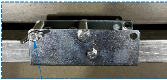
Wing-head bolt installed in first bolt hole
